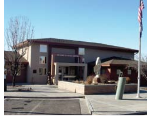
A 5 kilowatt photovoltaic system was installed at the Visitors Center.
