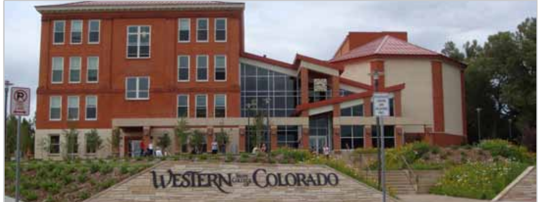
Under an energy savings performance contract (ESPC), Ameresco's team retrofitted lighting and water fixtures and replaced aging mechanical equipment and windows.
