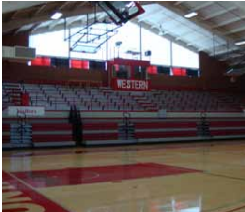
The lighting retrofit in the gym resulted in more evenly distributed light.
